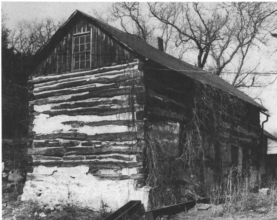
Figure 2. White oak log cabin near Middleton, WI, constructed around 1845 and never painted or finished.
