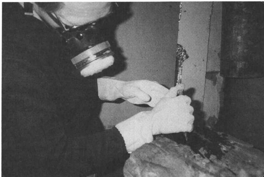
Figure 19. Conservator injecting friable surface with 22-gauge syringe.
