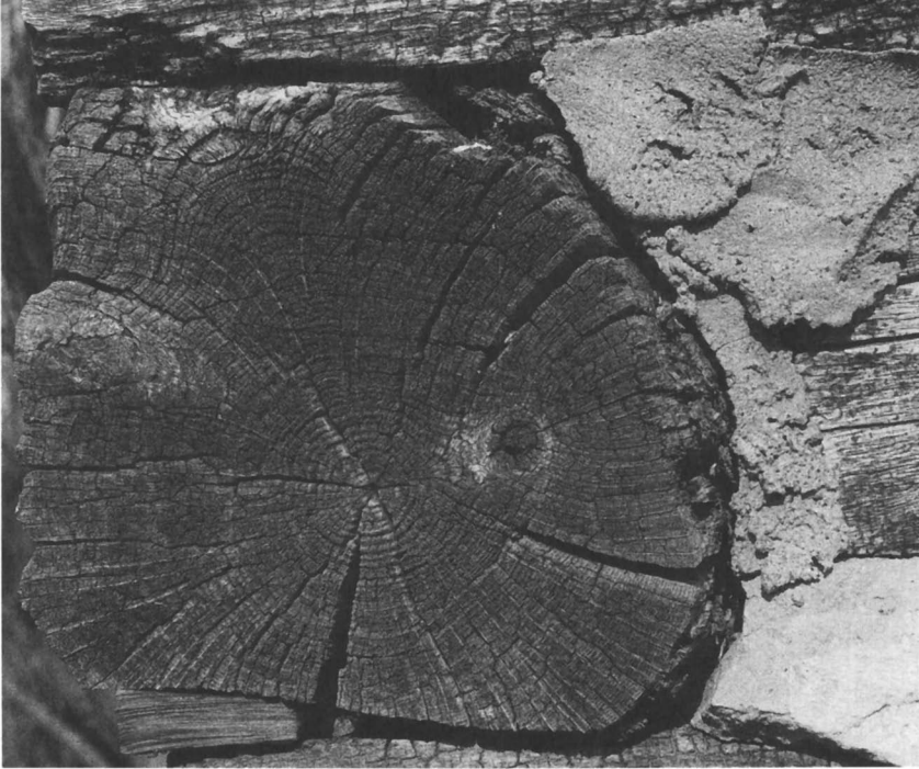
Figure 4. Close-up view of 140-year-old weathered white oak logs of house shown in Figure 2.
